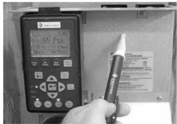
Figure 4. Easy ground check: Grounded
